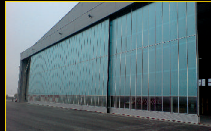
75 x 15 m door in Vilnius Intl. Airport
